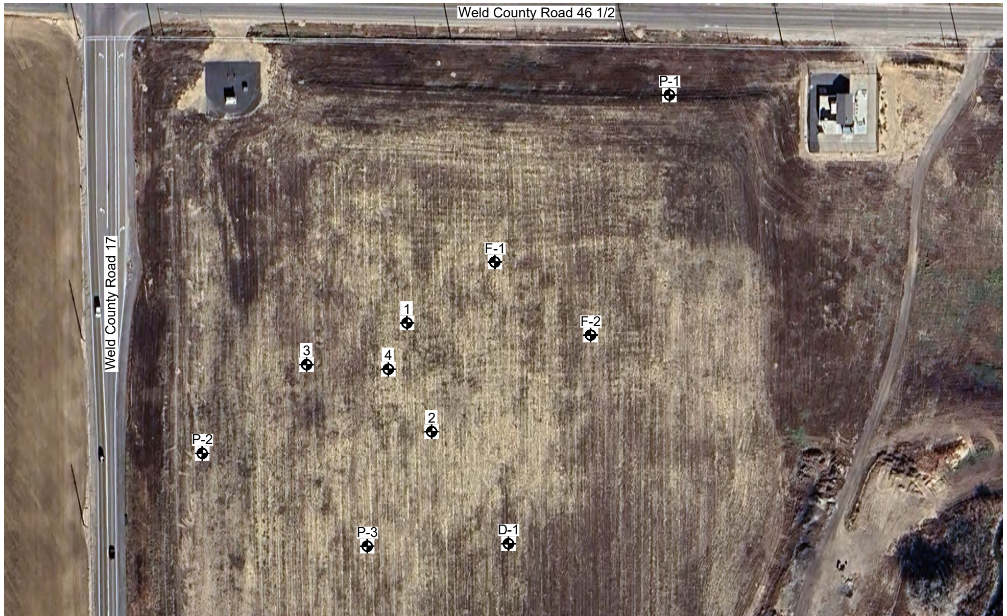
GOOGLE EARTH AERIAL IMAGE (11/12/2025)
